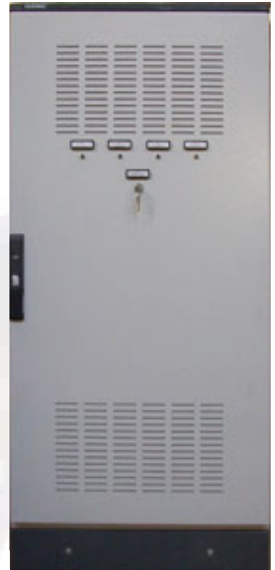
100kVA three-phase static switch
